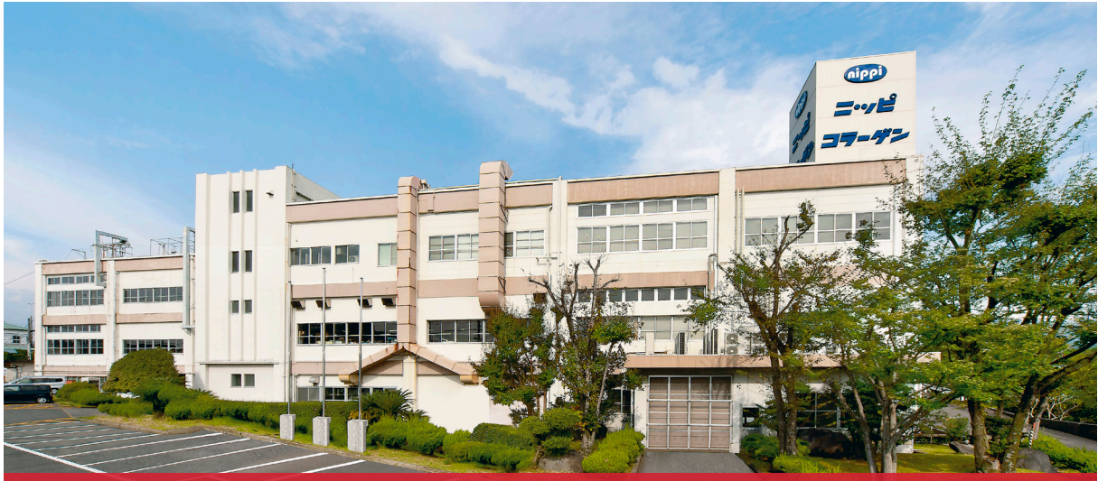
NIPPI PLANT, FUJINOMIYA, JAPAN
